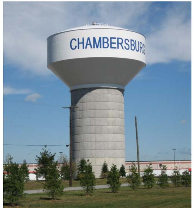
**Figure 4: Nitterhouse Drive Elevated Composite Tank**
