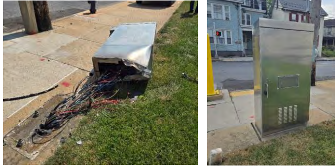
Replace Signal cabinet at Philadelphia Avenue and Commerce Street due to an MVA
