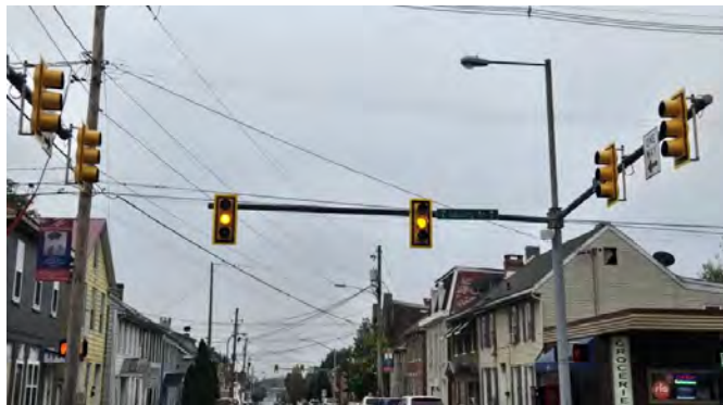
Signal head replacements at Main Street and Liberty Street- Hanging to modern signals with backplates
