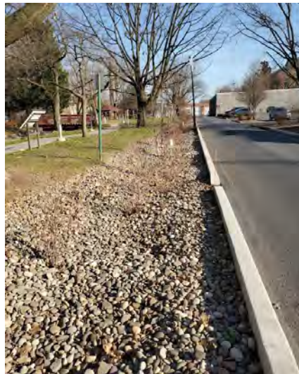
Rhodes Drive Borough-Owned Infiltration Area
