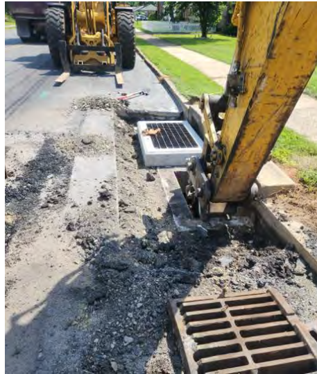
Storm Sewer Capital Improvements Project Associated with 2025 Street Improvements
