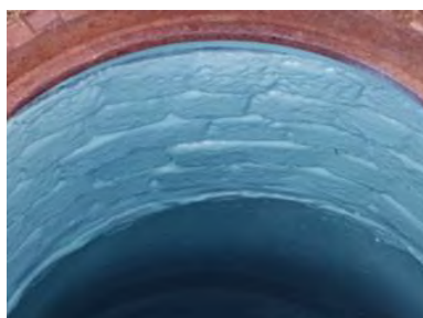
Manhole After Rehabilitation
