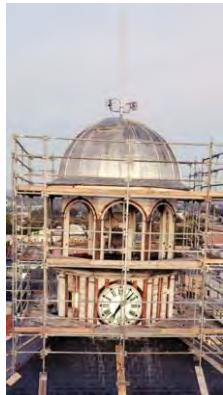
Clock Tower being restored in 2022
