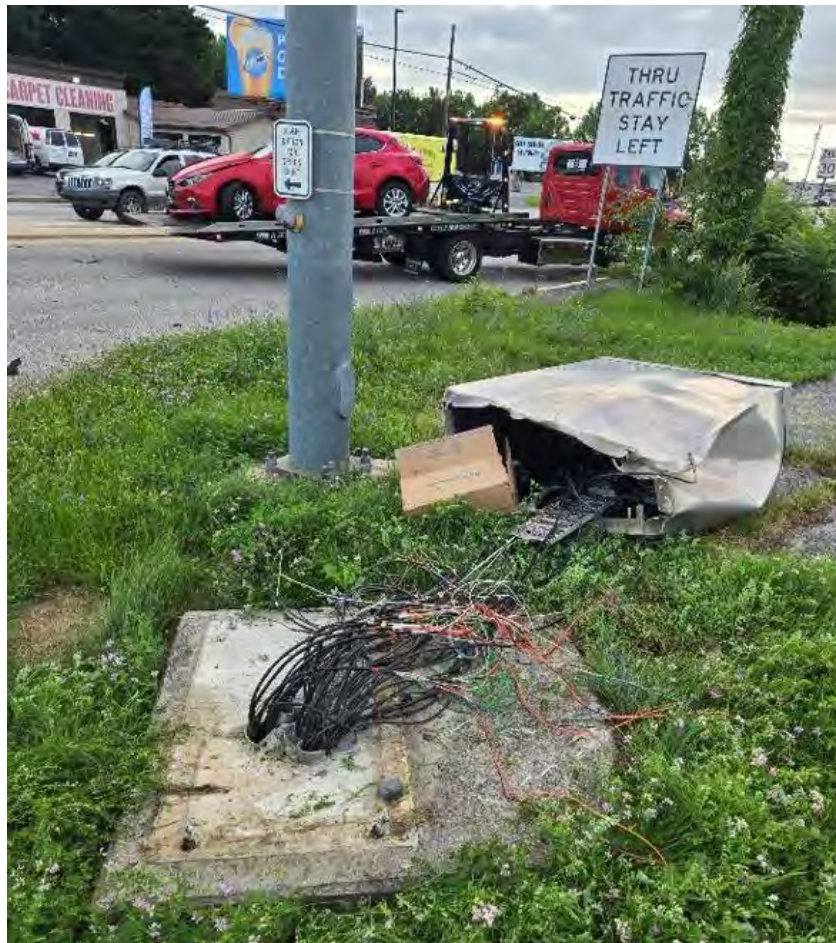
Replace Signal cabinet at LWE and Ragged Edge Road due to an MVA
