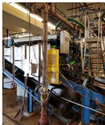
Aging Equipment – Belt Press
