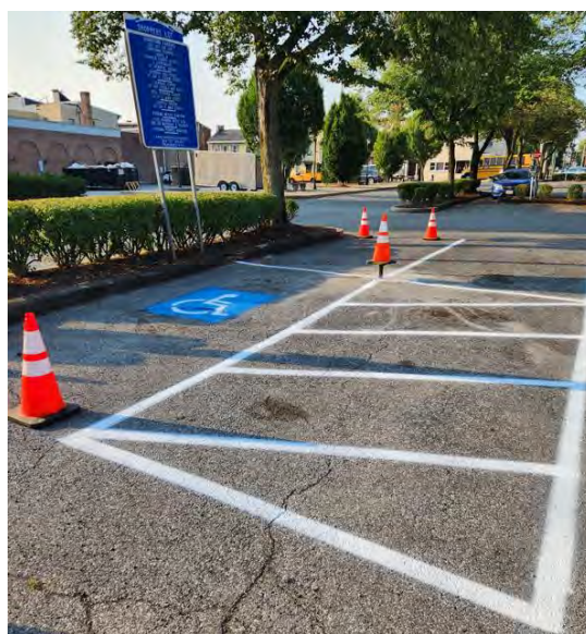
Installing Handicap Parking Stall
