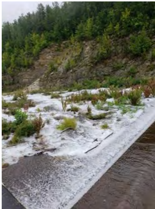
Long Pine Spillway – July 2018
