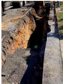
Sewer Main Installation
