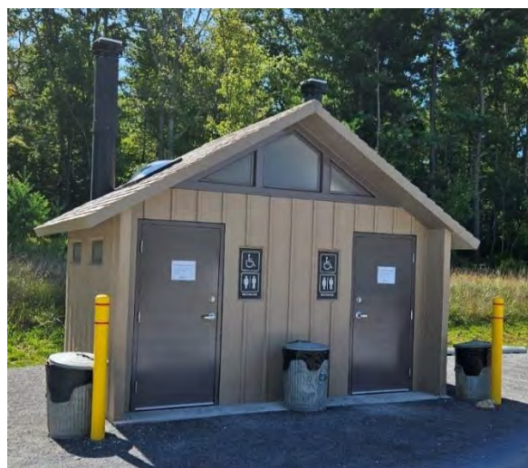
Long Pine CXT Restroom – Summer 2024
