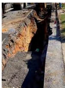
Sewer Main Installation
