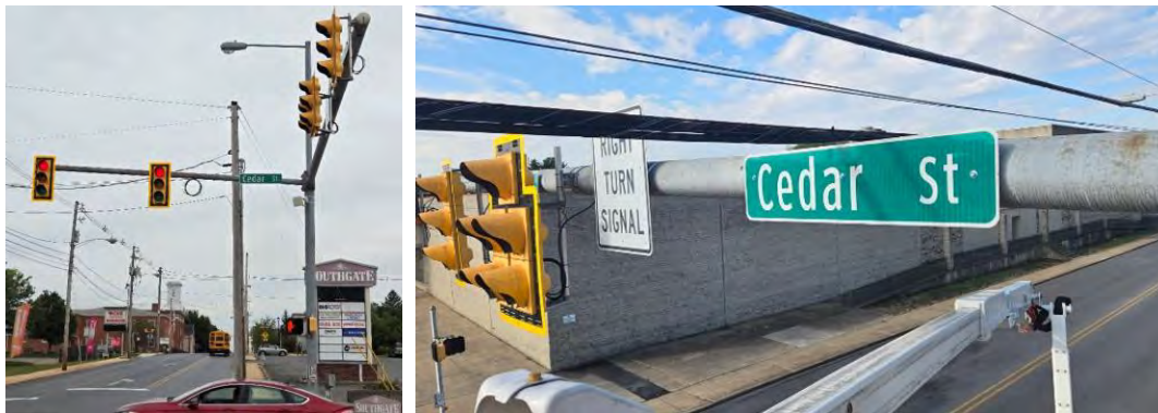
Installed signs to Rename Cedar Ave to Street per Council Directive
