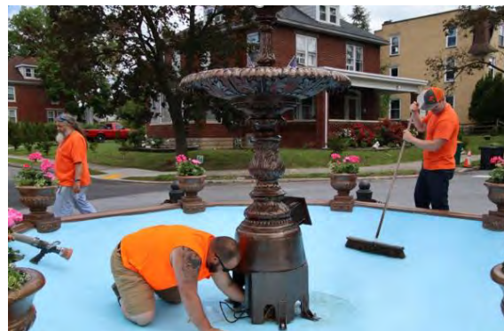
Resurfacing the Glenn Street Fountain
