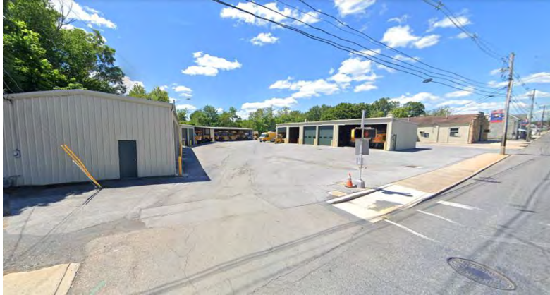
Loudon Street Public Works Facility
