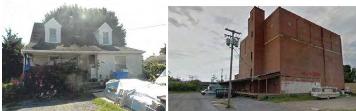
Former Buildings Demolished
