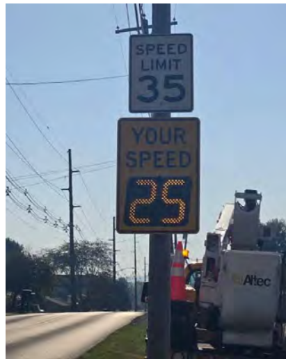
Replaced Radar Sign at Mill Road
