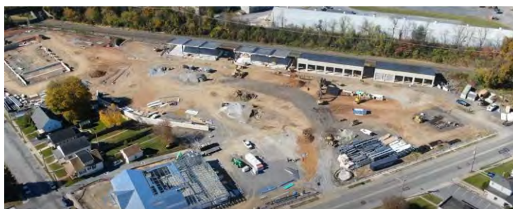
Construction Well Underway
