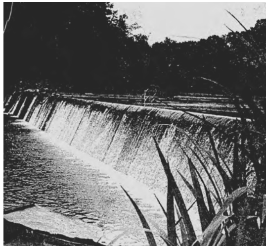
The Second Siloam Dam
