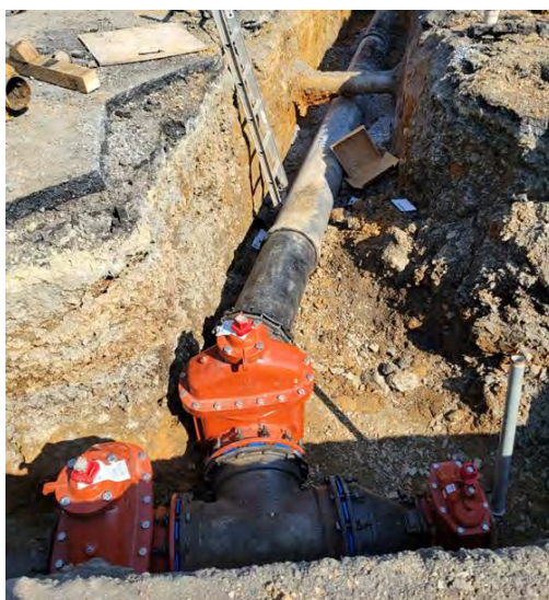
Chambers Street/Reservoir Hill Water Main Extension
