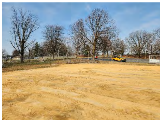
Demolition and repurposing of Nellie Fox Ball Field at Memorial Park
