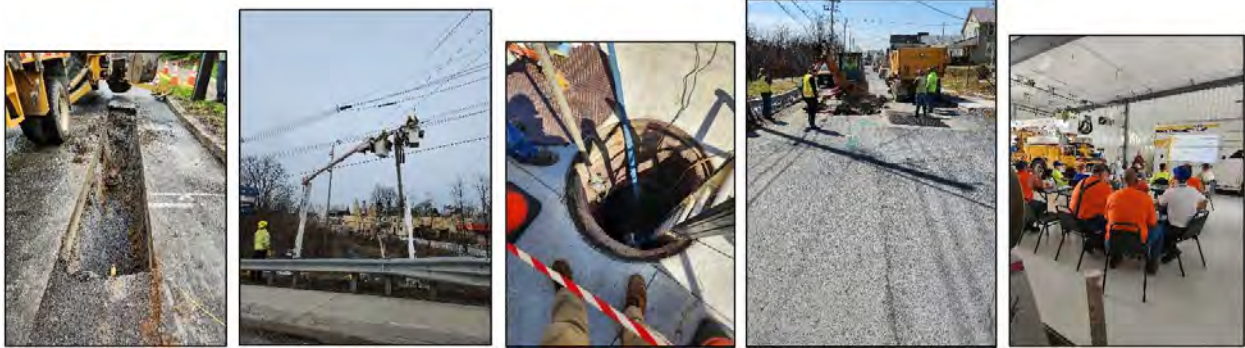
Pictured left to right: Gas Department- replacing a high-pressure line; Electric crew- working an accident location; Manhole with two employees inside doing confined space work; Highway Crew inspecting and repairing a sink hole; and Electric worker classroom training.
