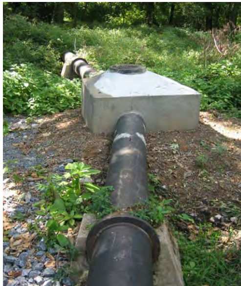
Falling Spring Sewer Interceptor
