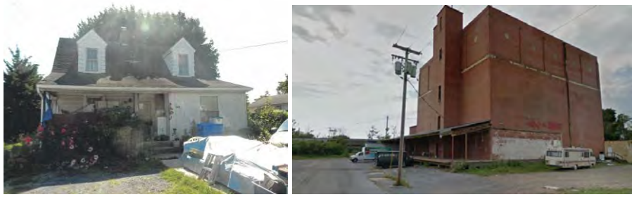
Former Buildings Demolished
