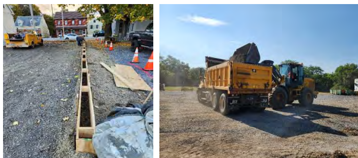
Highway Department Employees Building Curbs and Hauling Materials for Street Paving Projects
