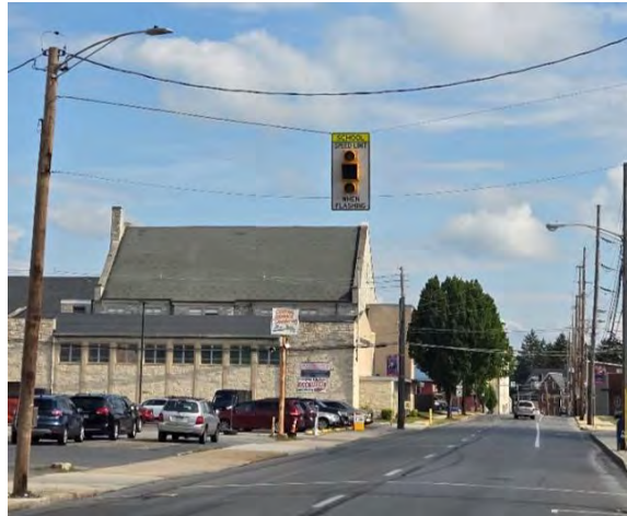
Relocated Corpus Christi School Zone flasher south to coincide with current school zone
