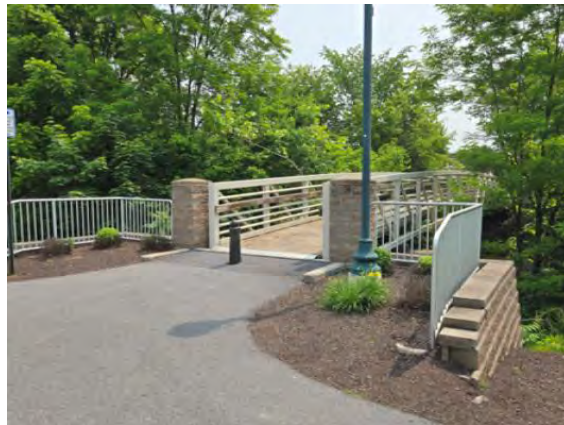
New bridge deck on the Chambers Fort Park Pedestrian Bridge
