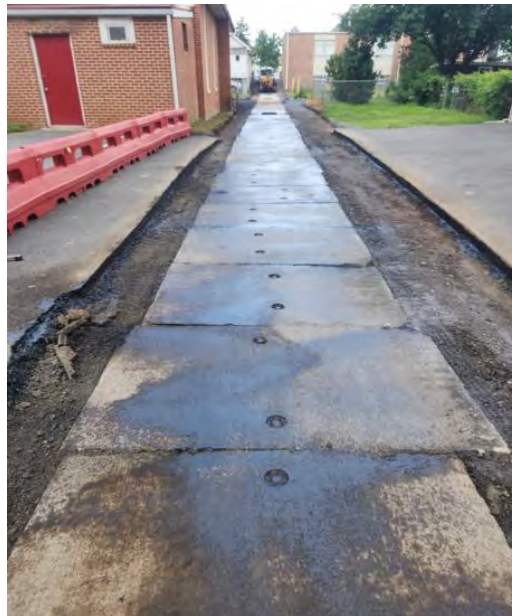
Clippinger Alley Box Culvert Repair Project
