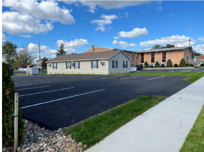
Renovated Bethel Assembly of God Church on Glenn Street
